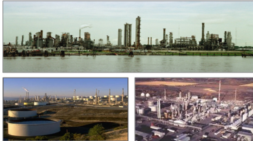
Figure 86. Examples of industrial facilities
