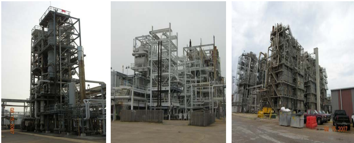
Figure 91. Examples of Open-Frame Structures
