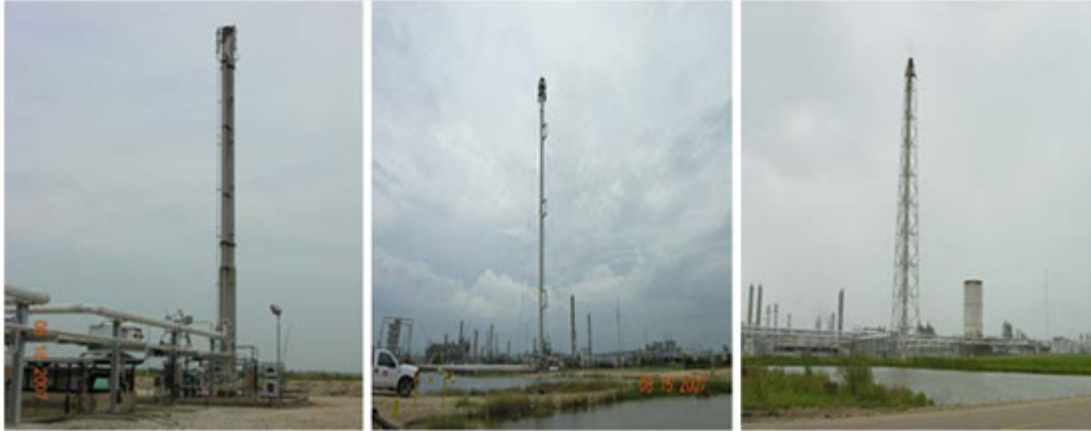
Figure 96. Examples of flare towers (left: freestanding flare, middle: guyed flare, and right: derrick-supported flare)
