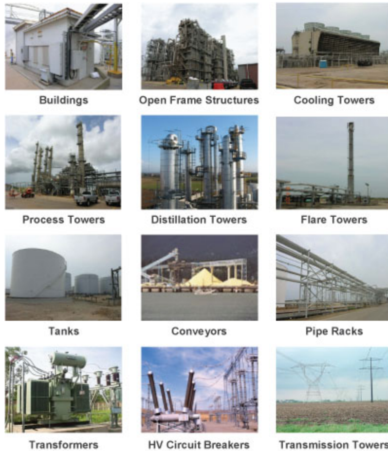
Figure 87. Examples of industrial facility components
